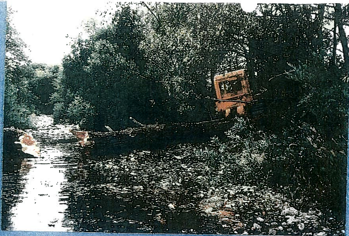
Plate 5. The dozer is procuring bank protection materials and skidding them across the river to a location accessible by the excavator and dump truck. The minimum disturbance to natural resources was a paramount concern during this phase.
