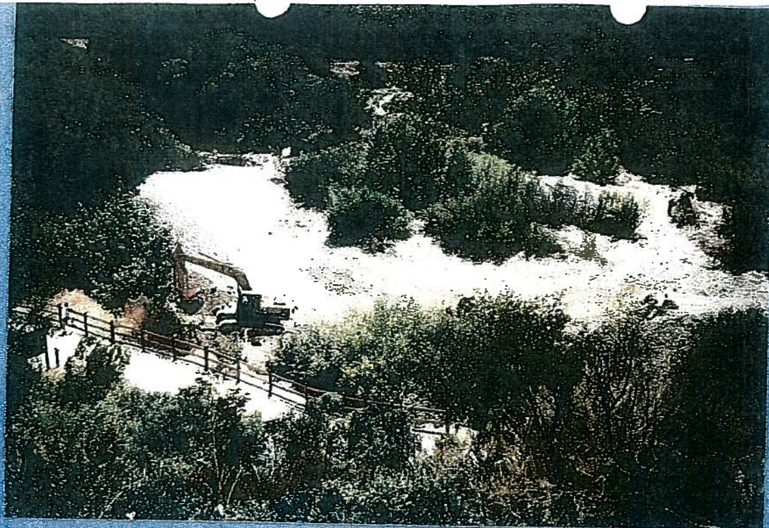
Plate 1. Overall view of the project site. The river has been diverted, it normally occupies the strip to the right and above the excavator. The floodplain is just above the active channel, with the terrace (Creamery meadow) at the top of the photo.
