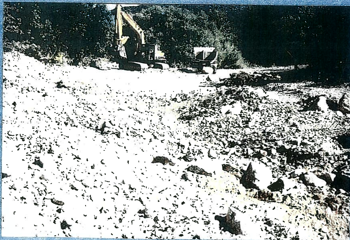
Plate 4. The straight reach of the project site has been roughed out. The convergence structures are being placed. The thalweg runs diagonally from left to right in the photo.
