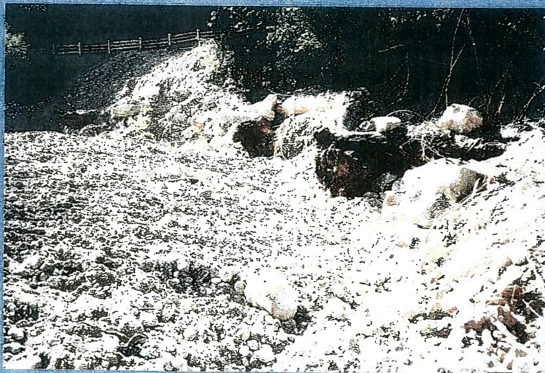
Plate 10. Now the site is ready for water. This is looking downstream. Note the orientation of the rootwads and the slope of the point bar. The point bar is the depositional feature on the left side of the photo. It is critical for dissipating the river's energy during high flow. It's shape and slope determine its effectiveness for this task.
