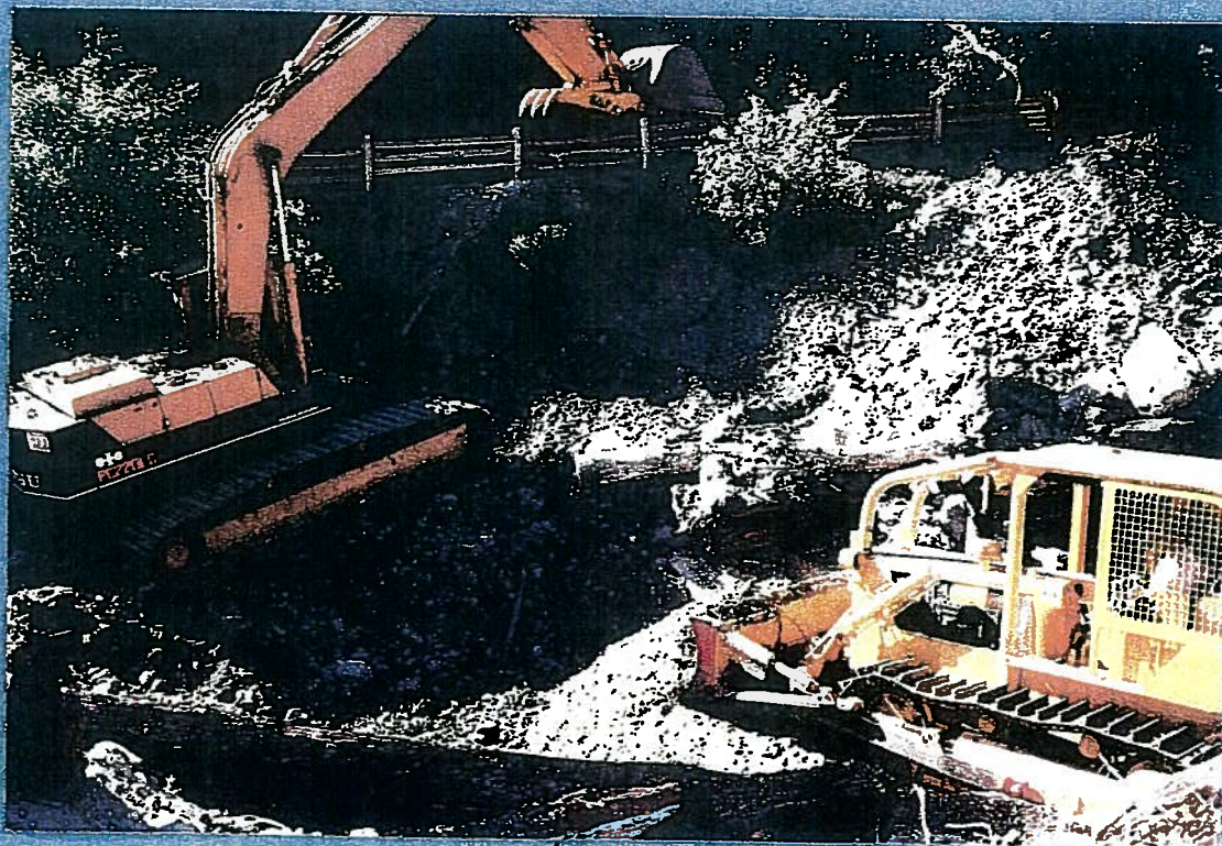
Plate 6. The excavator is backfilling the bank protection with free-draining channel material. The dozer is "feeding" the excavator to maximize efficiency. This material solves two problems- excess material in the active channel and bank failure from the "drawdown effect". The backfill is excellent for counter-bultrussing the slope.
